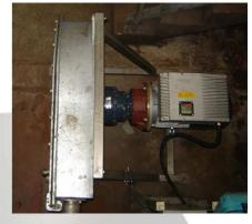
An L80 pump on an effluent application chosen due to its high flowrate and low power consumption. As well as saving on power, our low friction rollers dramatically reduce wear on the hose caused by the physical stretch and frictional heat from competitors fixed shoe designs, greatly extending overall hose life.
