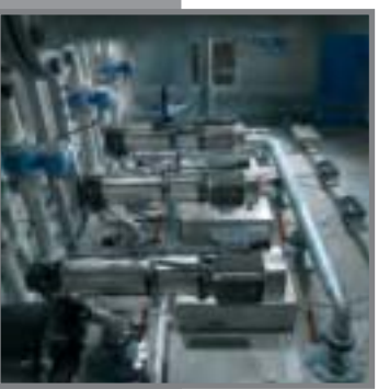
CR pumps in reliability test
